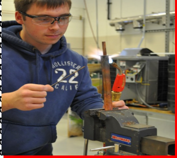
Greg Rogers works to fix a HVAC system at his Career Tech class.
