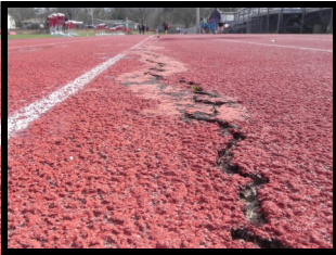
A picture of the current condition of the track.
